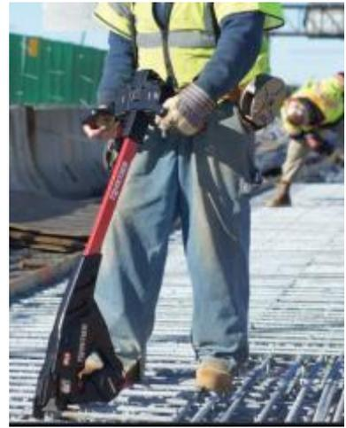
Binding of irons. Work at eye level. 5 times faster than a ligature done manually
