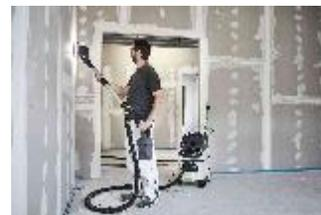
*Drywall sanding with lighting and vacuum. adjustable suction maintains its own weight on the wall or ceiling,*
