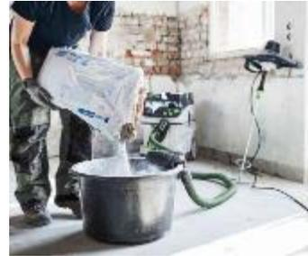
Mix any type of material without any dust. MX suction device, which simply attaches to the edge of the bucket, Flexible height adjustment device ErgoFix for an ergonomic posture
